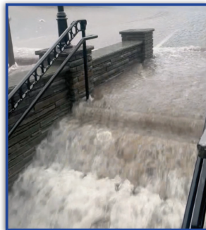
Rapid flooding near the Shalom Center
