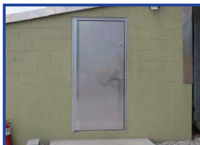
Mechanical Room Flood Door (PD-525)
