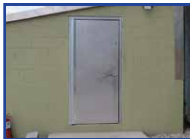
Mechanical Room Flood Door (PD-525)
