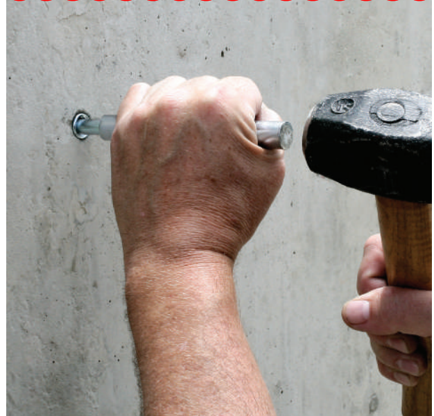
Anchor being set with hand setting tool.
