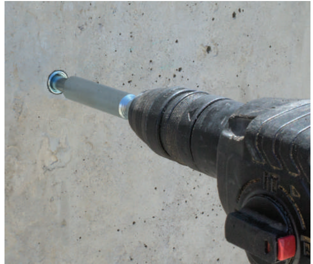
Anchor being set with SDS setting tool.
