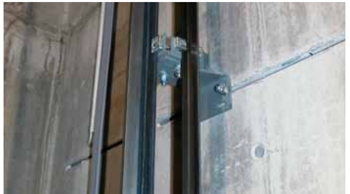
ELEVATOR CONNECTIONS
