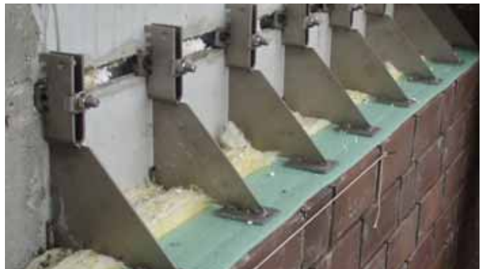
MASONRY CONNECTIONS
